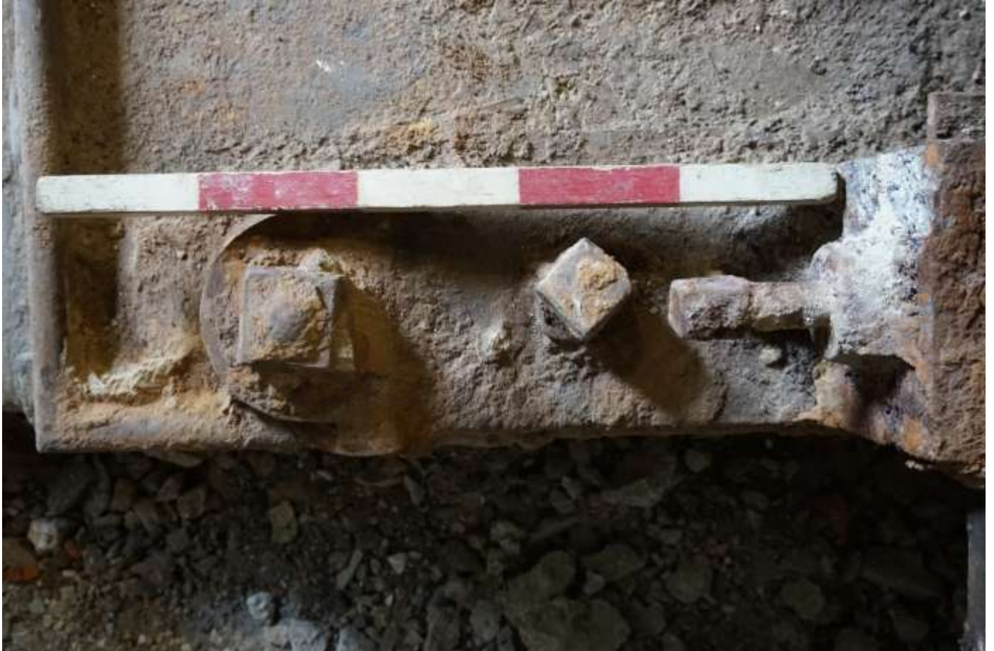
Plate 19: Bolt and nuts fixing iron plate with watershaft socket to the brick floor underneath
