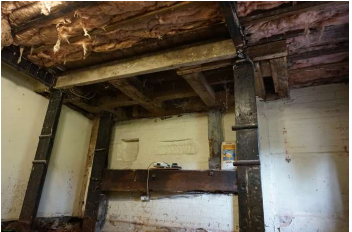
Plate 6: Looking west at the iron posts and beam supporting wooden beams and joists of upper floor. The Iron frame was harbouring gear mechanisms of the mill.
