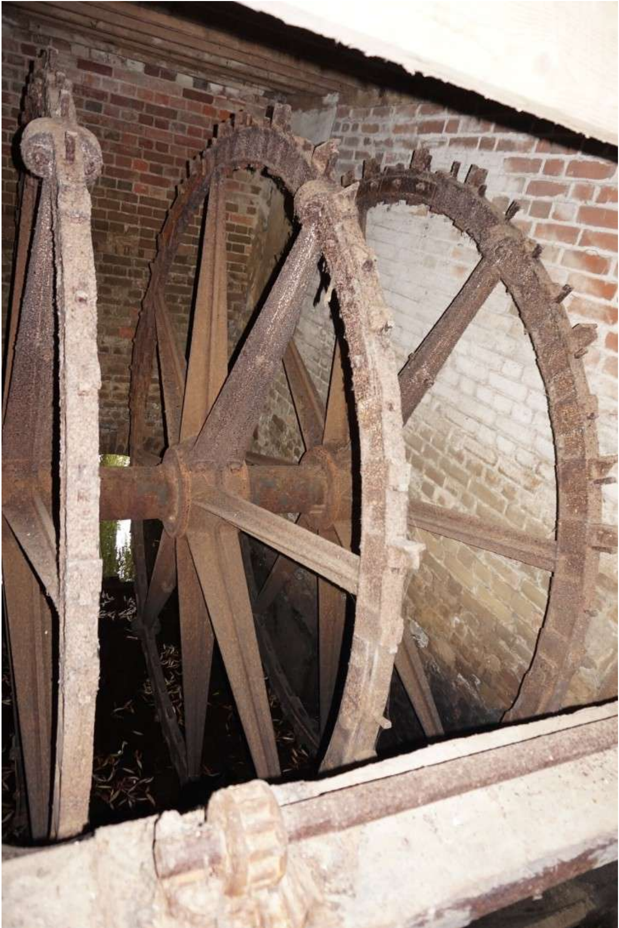
Plate 21: Looking north east at Water wheel. The water buckets were removed some time ago.
