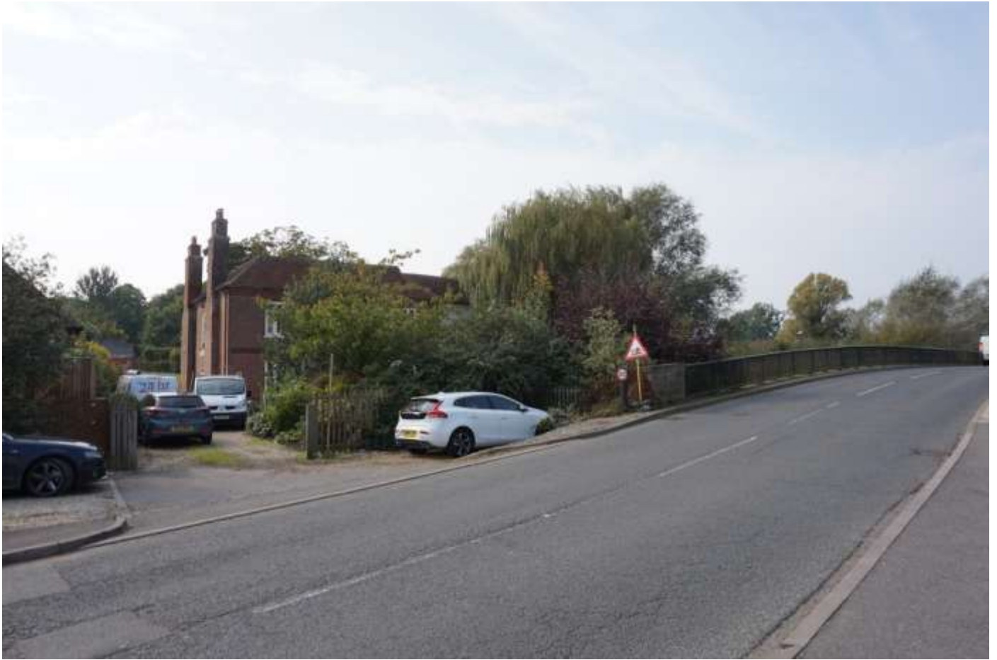
Plate 1: Looking south west at the Mill house.
