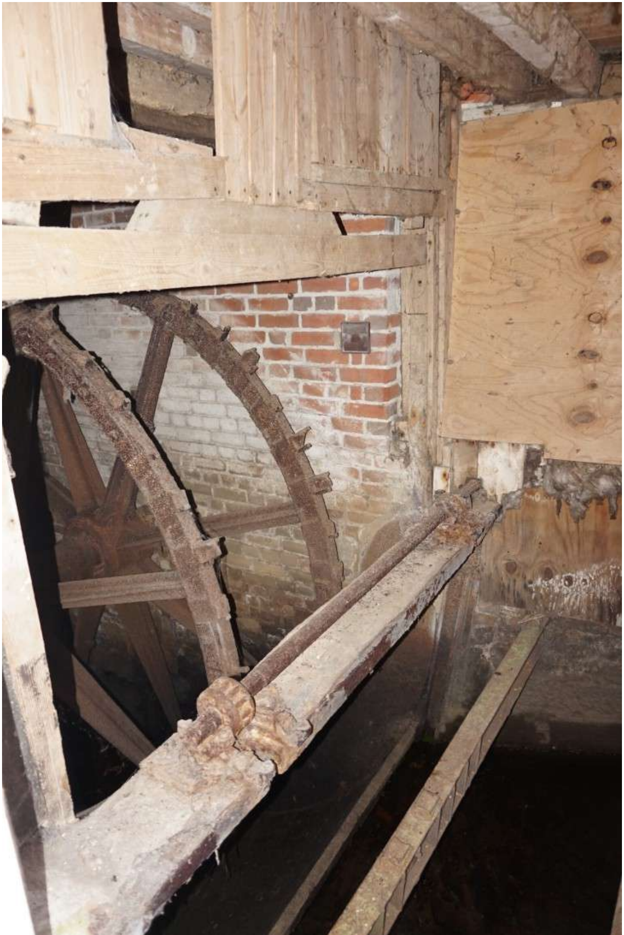
Plate 20: Looking east at remains of dam mechanism at the end of pentrough visible to the right.
