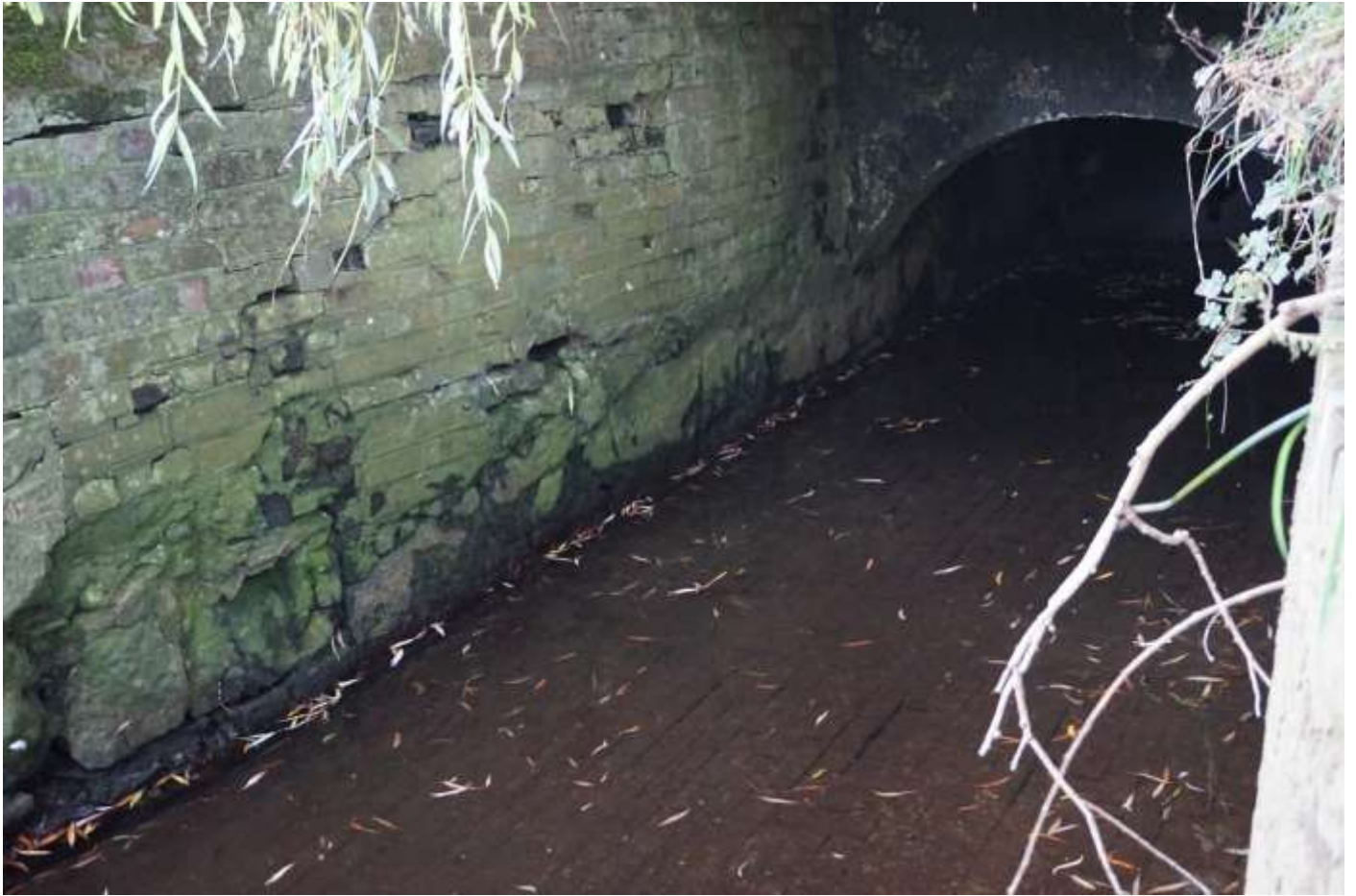
Plate 22: Looking south at water channel exit from Wheel room.
