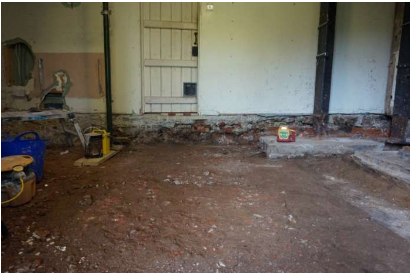
Plate 8: Looking south at the section through concrete floor overlaying levelling rubble deposit and wall remains.
