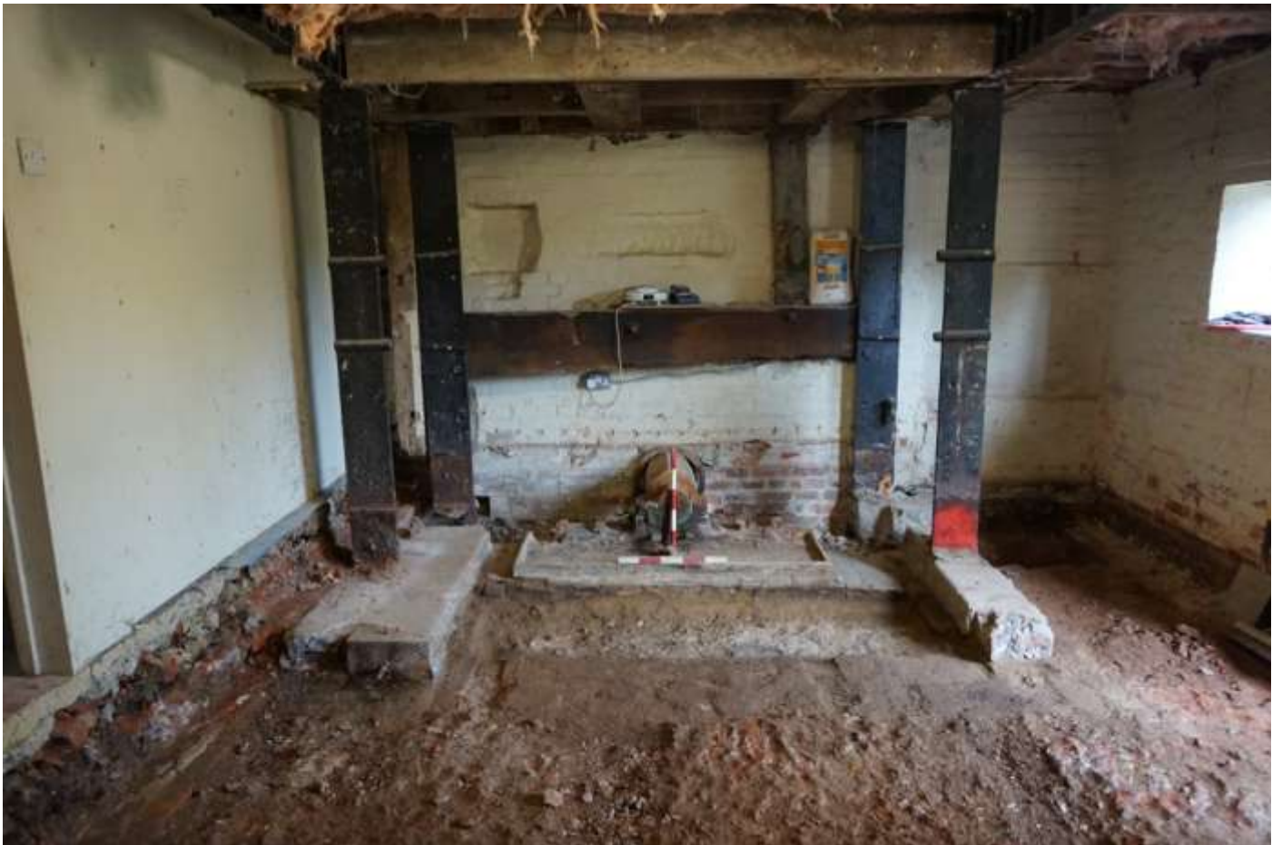
Plate 13: Looking west at iron post supporting beams and joist of upper floor. The iron posts were harbouring gear mechanisms of the mill
