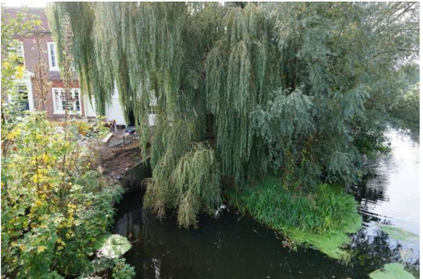
Plate 2: Looking south at the Mill house.
