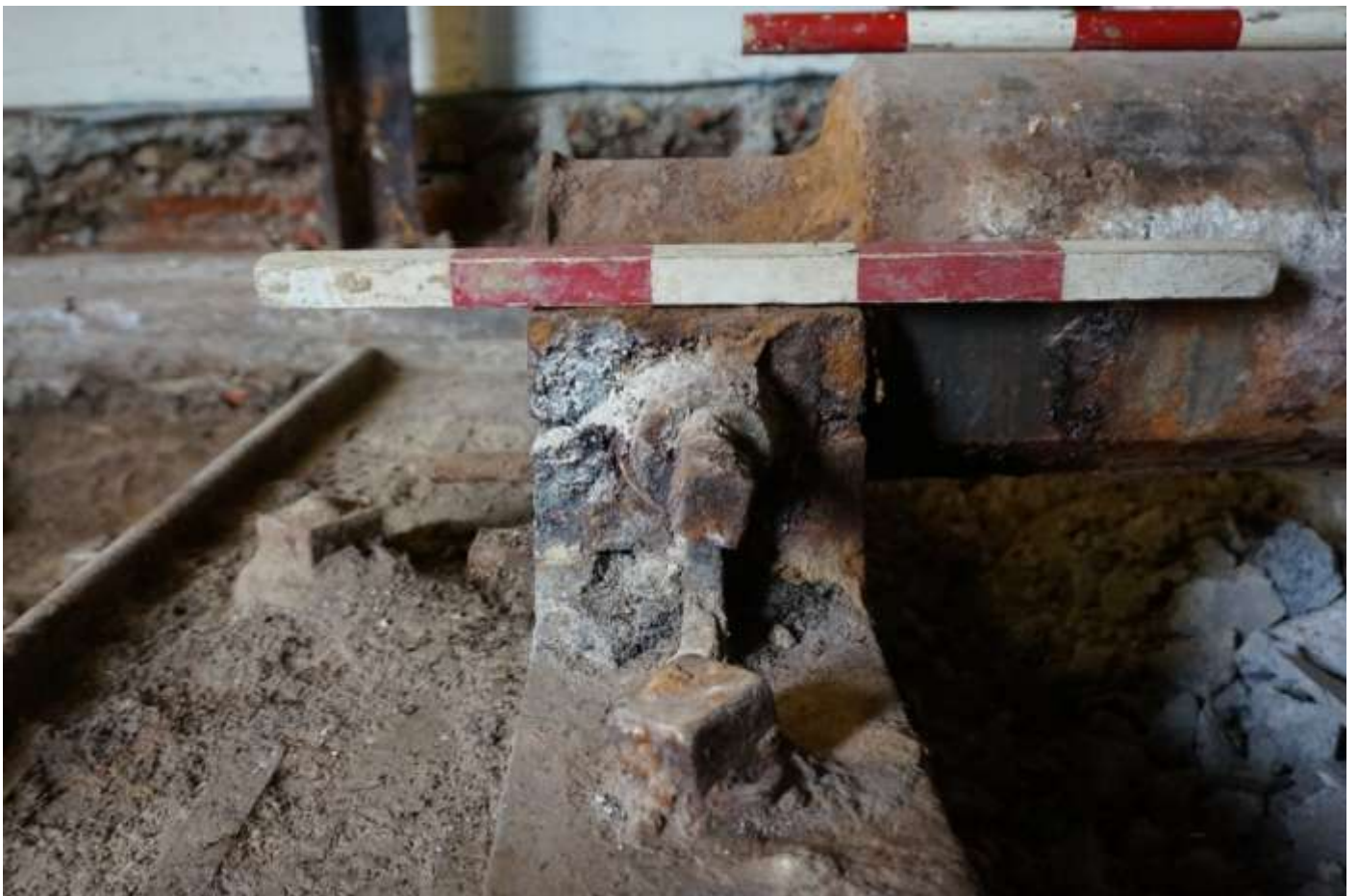
Plate 17: Side view of watershaft socket
