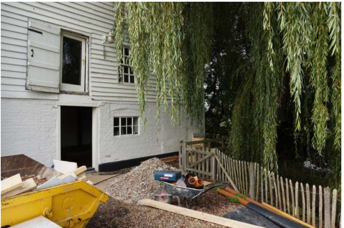
Plate 4: Looking west at the corner of the Mill house
