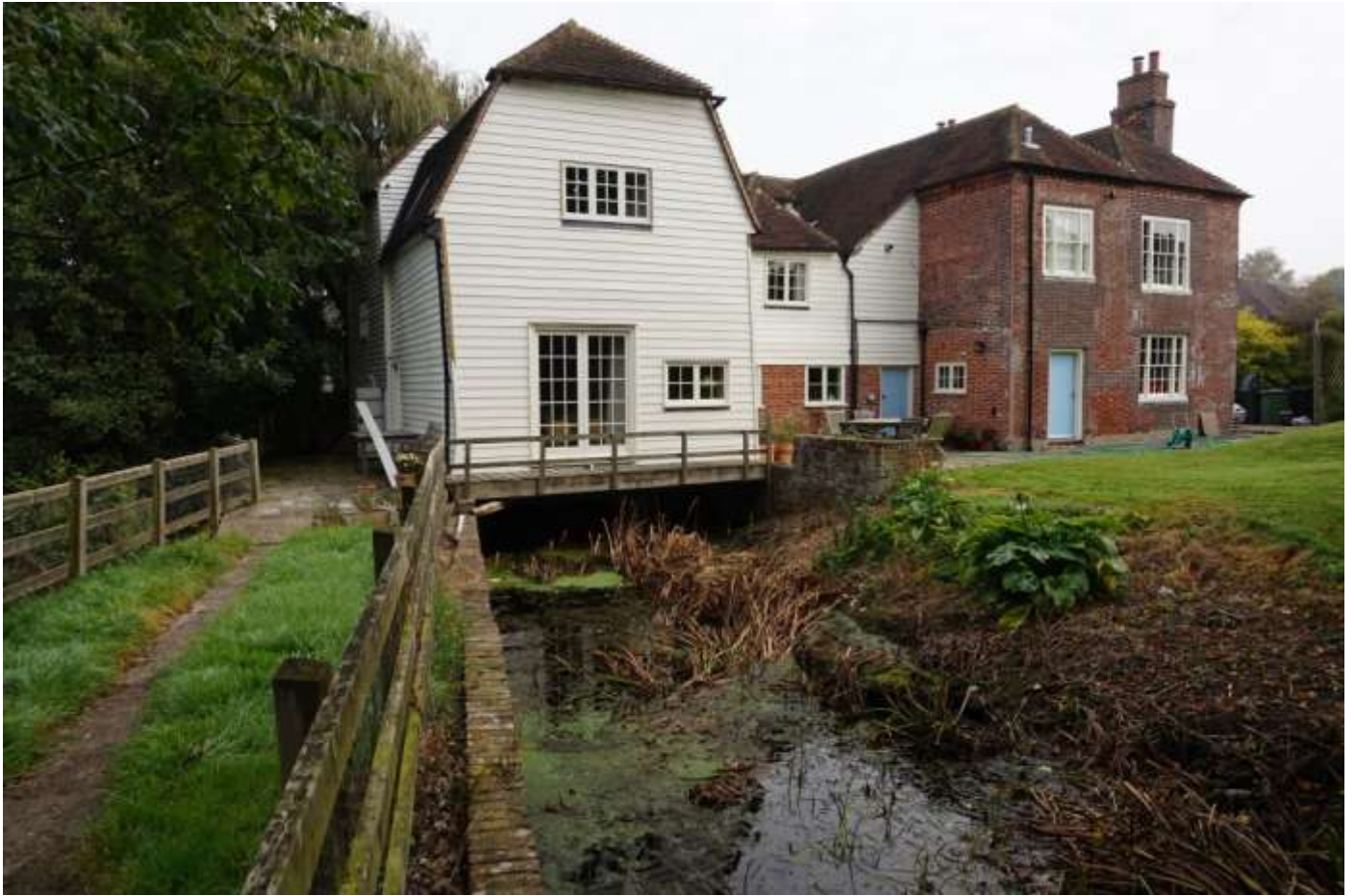
Plate 3: Looking north east back of the Mill house
