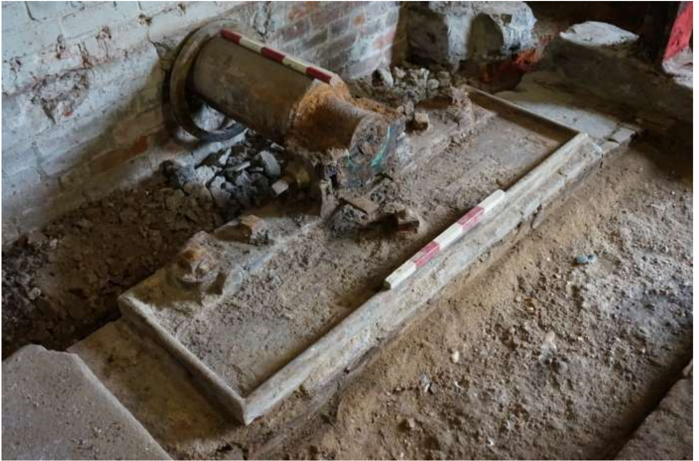
Plate 14: Looking north west at iron plate with watershaft socket and watershaft.
