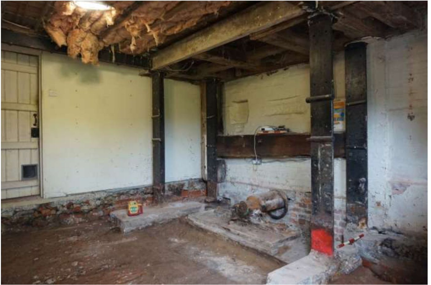
Plate 5: Looking south west at iron frame and wheel shaft.
