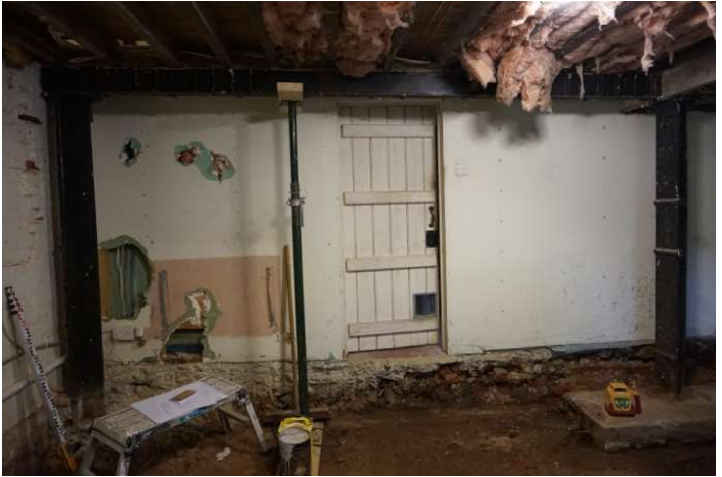
Plate 7: Looking south at the iron posts and beam supporting wooden beams and joists of upper floor.
