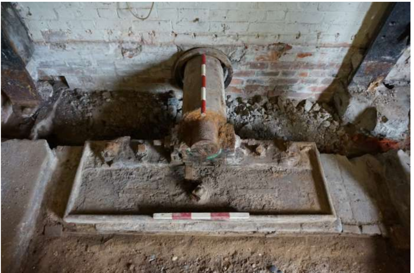
Plate 15: looking west at iron plate with watershaft socket and watershaft.
