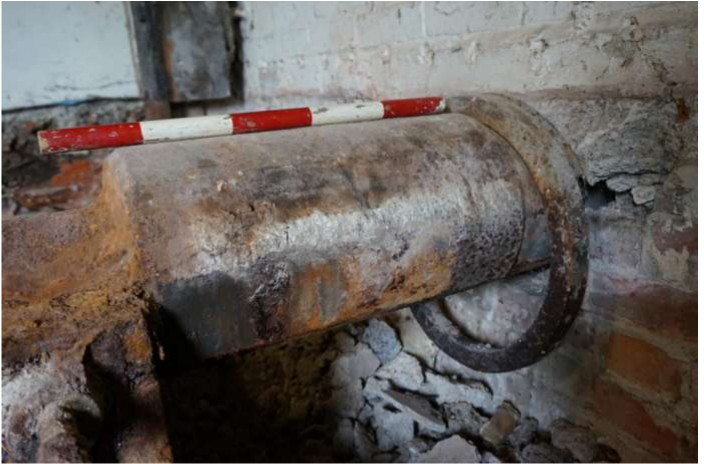
Plate 16: Pitwheel end of watershaft
