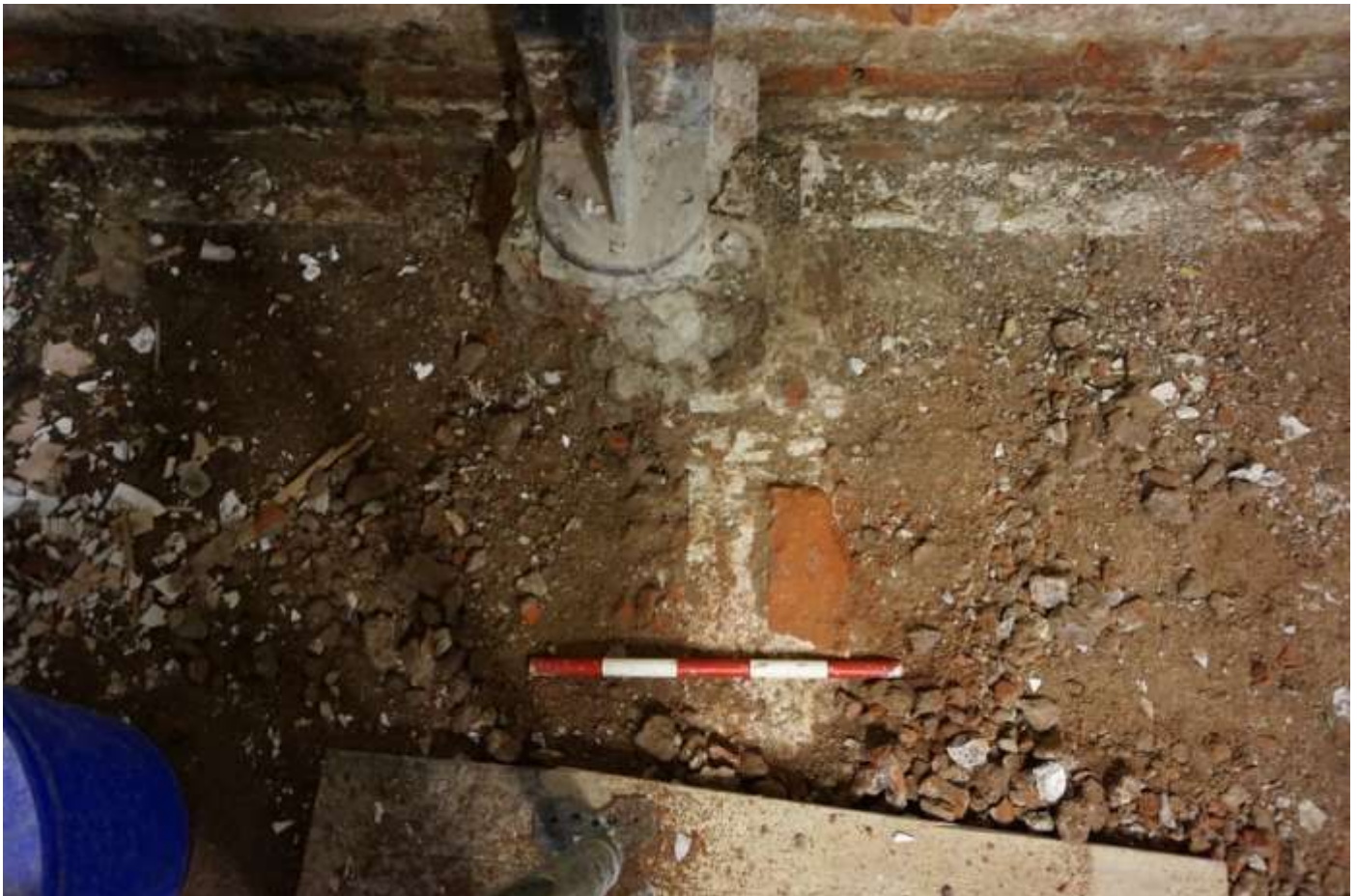
Plate 10: Looking east at brick wall foundation.
